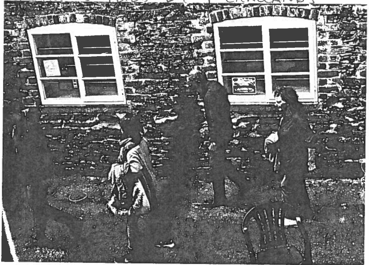
A party of four customers leaves by the emergency exit from the bar in June 2018. On other occasions customers have used this route while carrying drinks and/or smoking. The frequency of use has increased recently.
